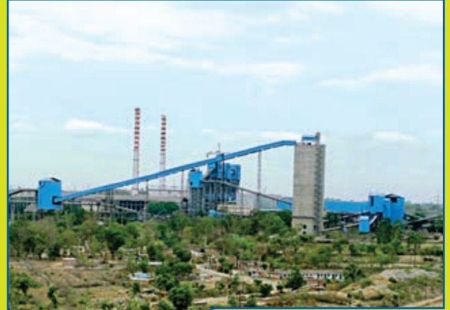
Captive Power Plant, Churk (U.P.)
