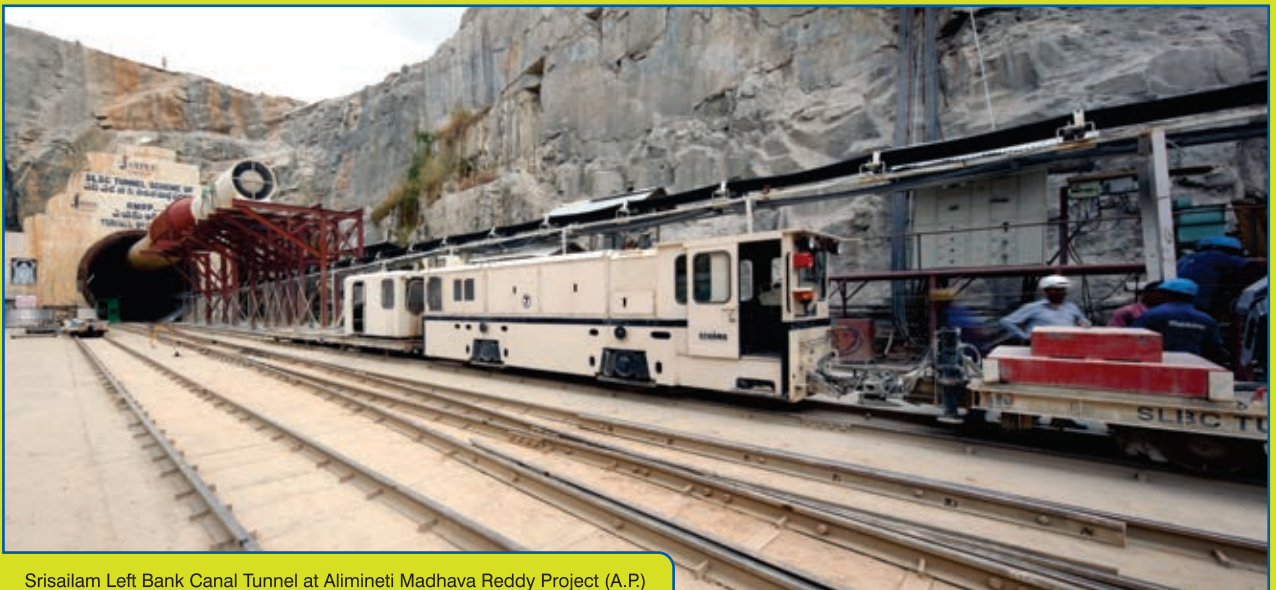
Srisailem Left Bank Canal Tunnel at Alimineti Madhava Reddy Project (A.P.)
