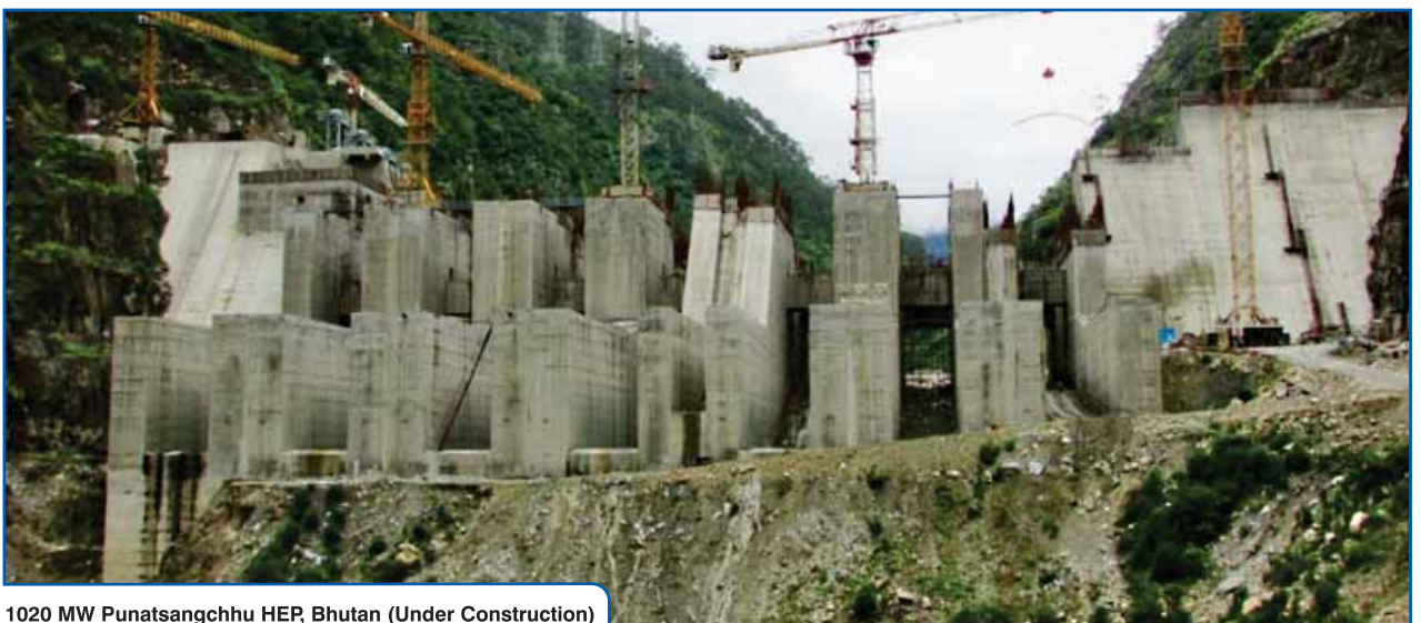
1020 MW Punatsangchu HEP, Bhutan (Under Construction)
