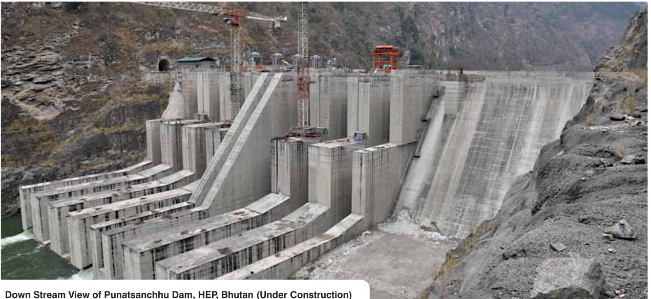
Down Stream View of Punatsanchhu Dam, HEP, Bhutan (Under Construction)
