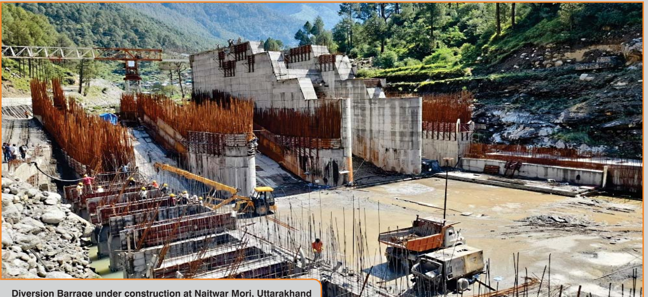
Diversion Barrage under construction at Naitwar Mori, Uttarakhand
