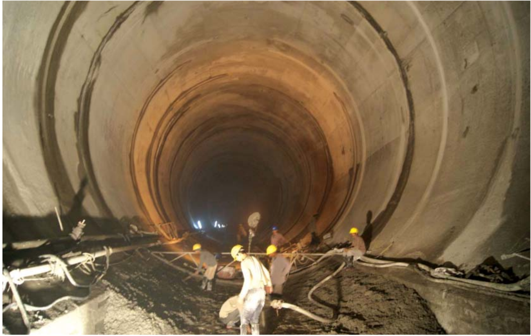
Head Race Tunnel Work in Progress at 1000 MW Karcham Wangtoo H.E.P., Himachal Pradesh
