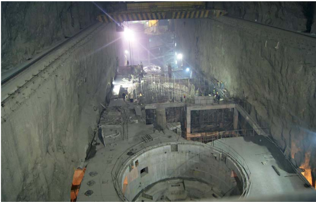
Machine Hall Under Construction at 1000 MW Karcham Wangtoo H.E.P., Himachal Pradesh
