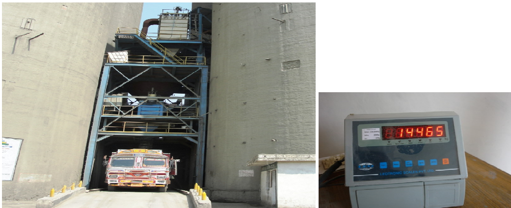
Automatic Cement Bulk Loading System
